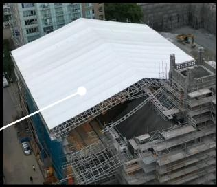
Climate protection is at the forefront of our design philosophy. Our Roof System is engineered to withstand a variety of heavy weather conditions, including heavy rain, strong winds, and even large snow loads. The high-quality keder tarps used in our system offer superior waterproofing and UV resistance, ensuring that your valuable assets and personnel stay protected in any climate.
