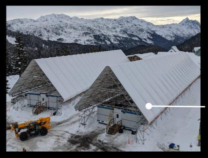
This image shows the roof structure that protected Brock Hall at the University of British Columbia (UBC) during its renovation phase. The scaffold provided a secure and accessible platform for workers, while the roof ensured the site was protected from adverse weather throughout the duration of the project.
